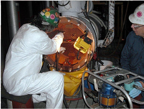
Figure 9 - Individual Tube Hydrotesting System
